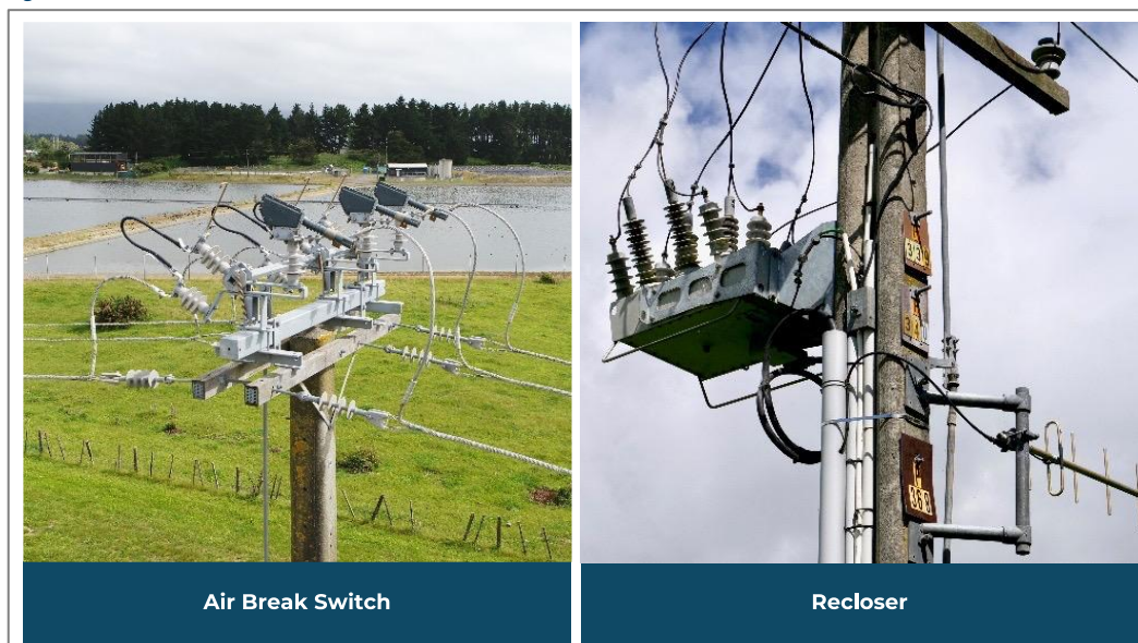
Figure 148: Pole-Mounted Switches
