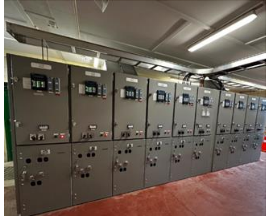
11kV switchgear at Levin East zone substation
