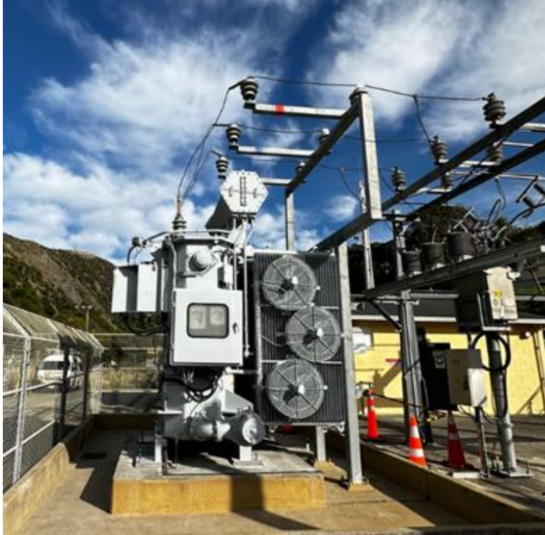
Paekākāriki power transformer replacement
