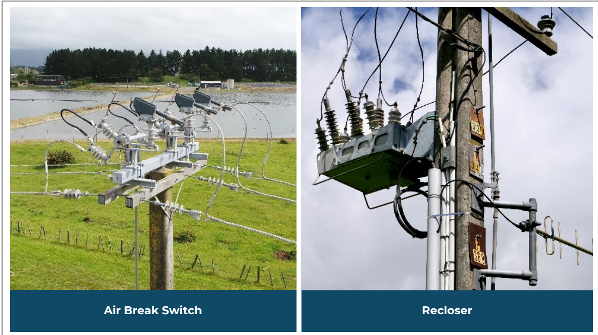
Figure 147: Pole-Mounted Switches
