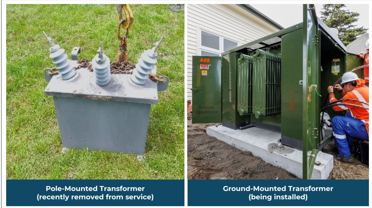
Figure 151: Transformers
