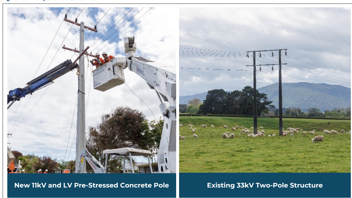
Figure 135: Example of Pole Structures
