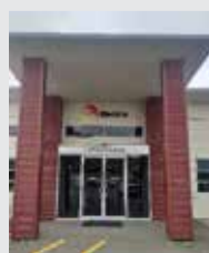
The current Paraparaumu depot
