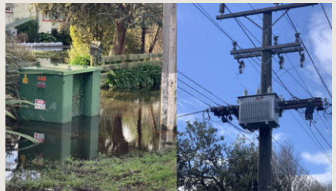
Union Street, Foxton: our ground-mounted transformer was subjected to flooding during heavy storms so it was replaced with a pole-mounted transformer
