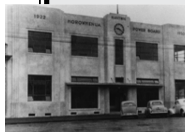
The original head office building in Queen St Levin.
