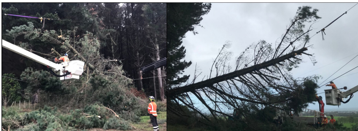
Figure 7-7: June 2022 Tree fallen on Mangahao-Levin East 33kV line during adverse weather
