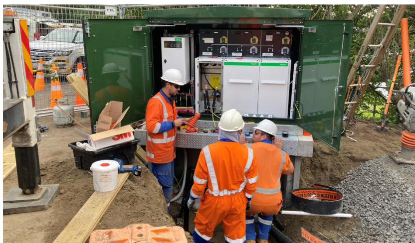
Figure 8-12: Installation of Golf Road automation switchgear in July 2021
