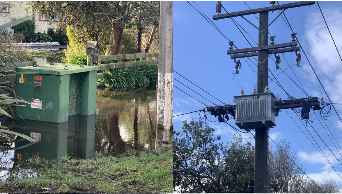
Figure 7-9: Foxton, Union Street Transformer C160: (a) Ground-mount subjected to flooding during heavy storms; (b) Pole-mount replacement.
