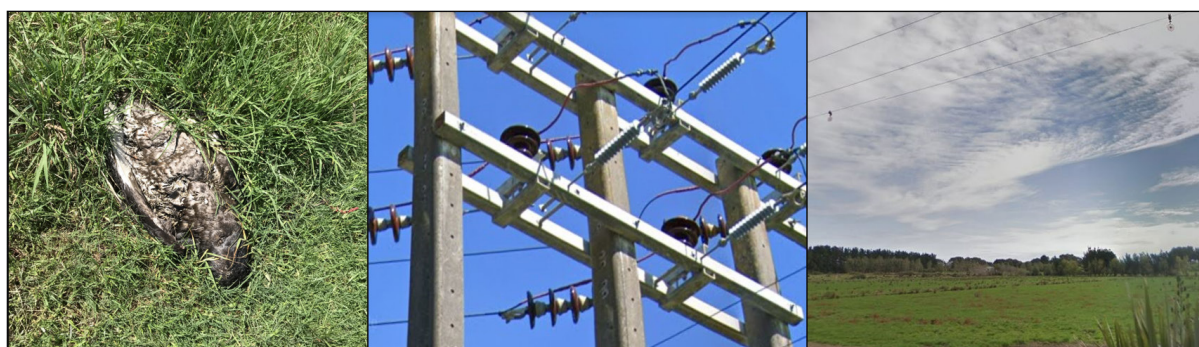
Figure 8-16: (a) Bird strikes causing faults on Levin West-Foxton 33kV line; (b) HV taping at 33kV conductors; (c) Bird divertors along Waihou Road line.
