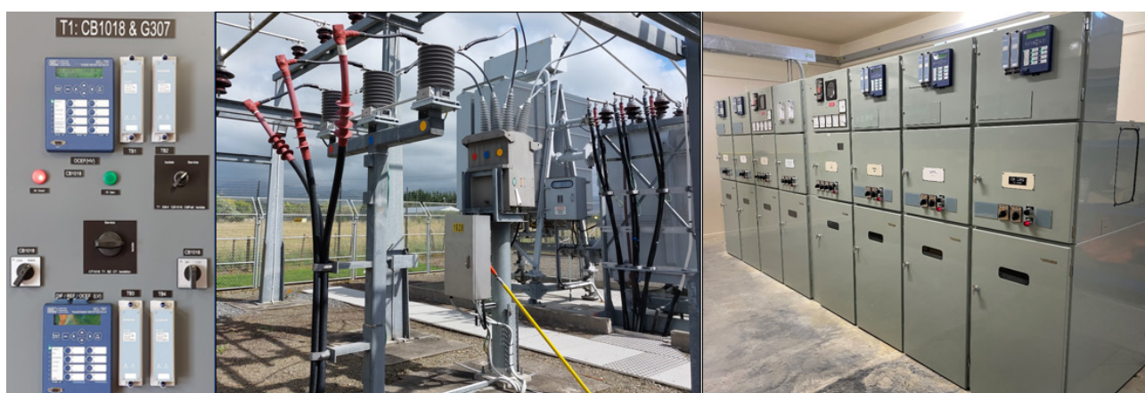
Figure 4-10: (a) Levin East transformer protection upgrade; (b) New outdoor 33kV CTs at Levin East; (c) Ōtaki Substation 11kV feeder protection upgrade.
