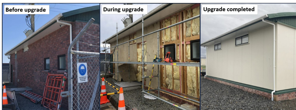
Figure 5-22: Ōtaki Substation seismic upgrade completed in May 2022
