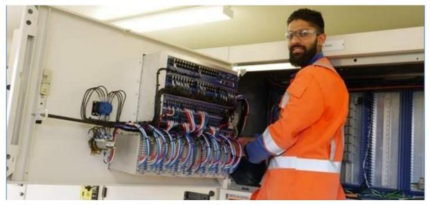
Figure 6-16: Installation of SEL-487B relay for Shannon Substation 33kV busbar protection upgrade
