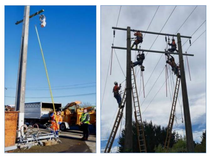
Figure 7-1: (a) Training on S&C TripSaver operations; (b) Maintenance on ex-Transpower 33kV H-pole structure
