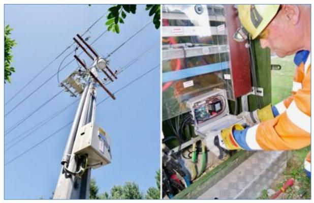
Figure 6-12: (a) 11kV Entec recloser switchgear (b) Power quality monitoring at transformer panel
