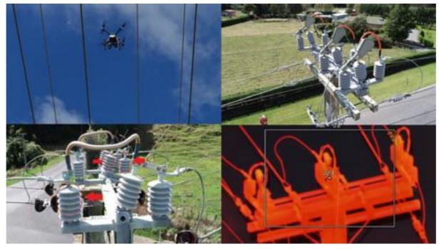
Figure 6-15: Continued improvement of condition-based risk monitoring of assets using UAV drone inspections and thermal imaging
