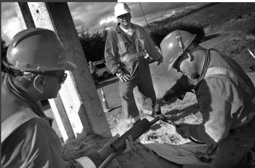
Network cable jointing
