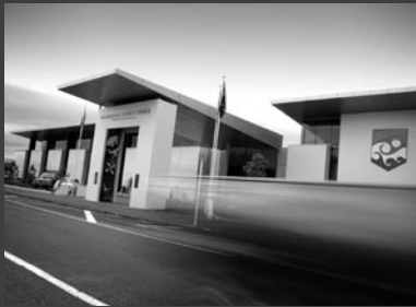
Horowhenua District Council building
