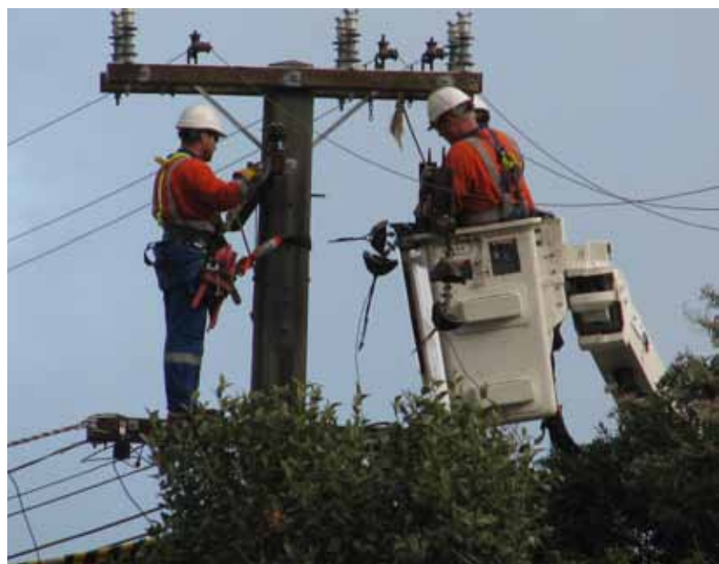
Reconductoring Forest Road, Paraparaumu
