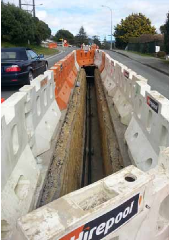
Construction of 33kV cable Ruapehu Street, Paraparaumu
