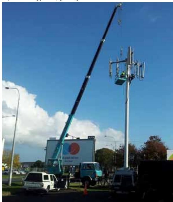
SkyComm riggers upgrading a Vodafone Microwave Link
